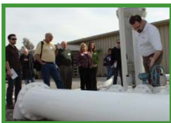
The AGTAC Center provided the opportunity to learn about water efficient pumps.
